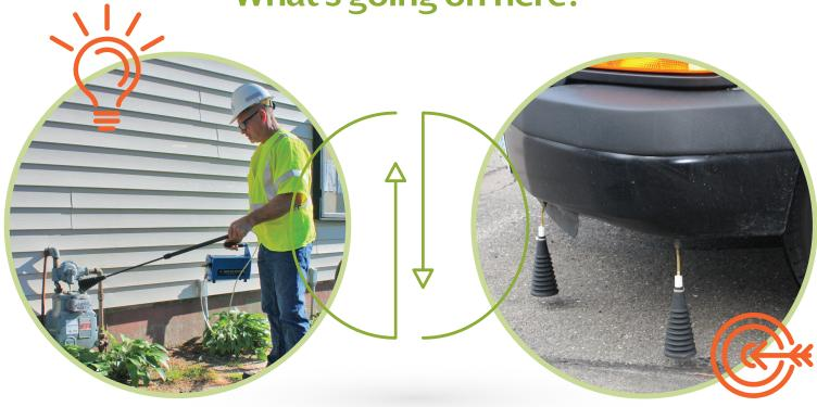
Trained MNG personnel have a variety of tools that help them locate and repair natural gas leaks. These include handheld detectors and even specialized "sniffer" trucks that ferret out roadside leaks.
